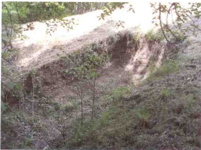
Washout halfway up the bank
