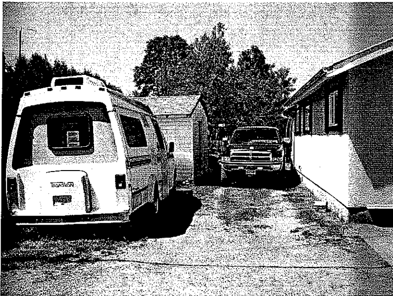
Photo 1: This photo shows the location of the proposed addition and shed to be removed.
