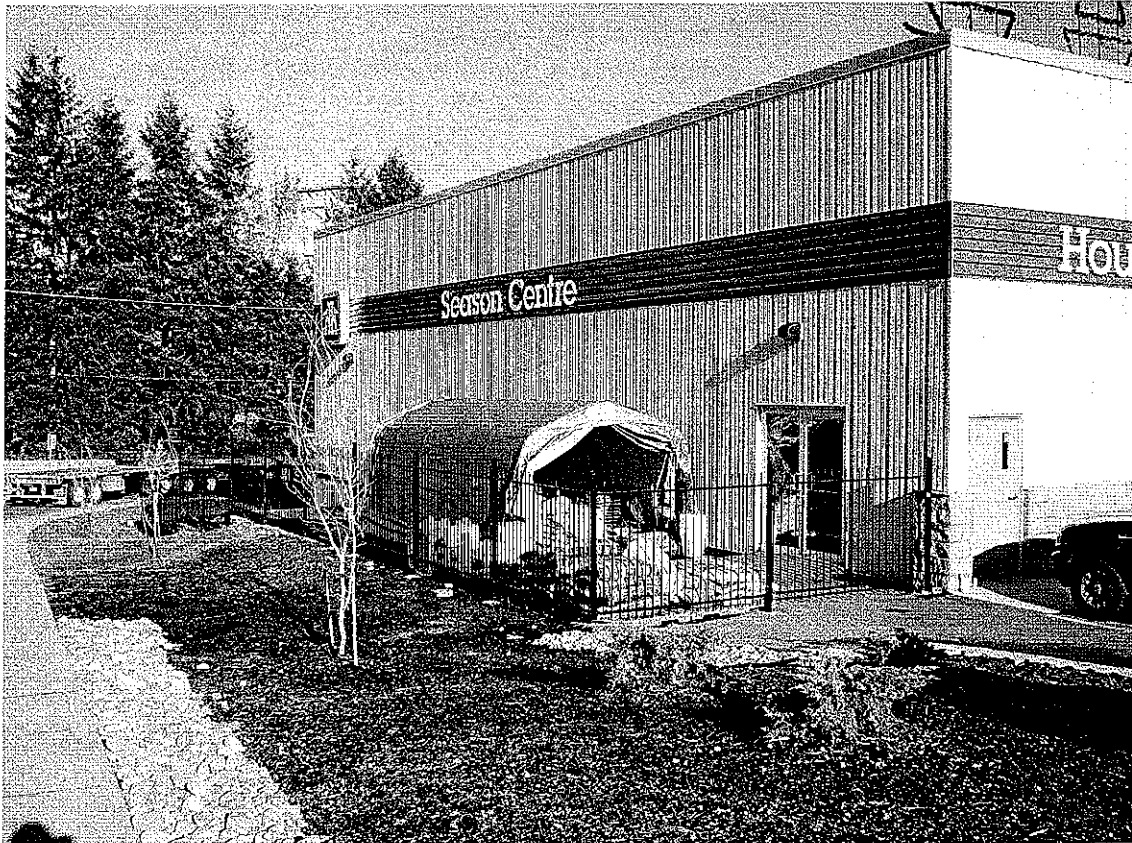
PHOTO 1: The proposed greenhouse would be located on the north side of the existing Home Hardware building. The black fencing shown is located on the property line and would be removed.
