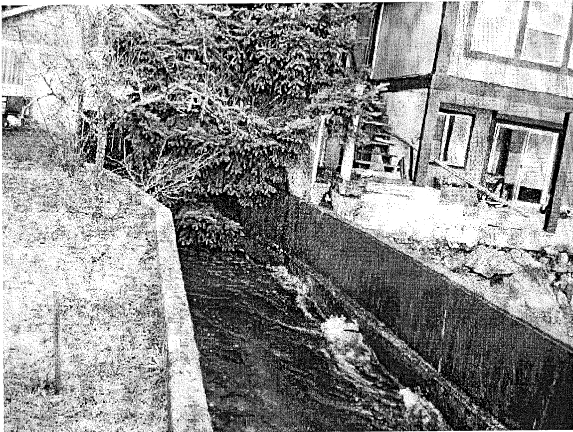
Photo 1: Russell Creek Concrete Channel Spillway adjacent to 341 Chemainus Road
