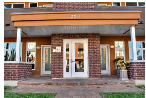
Example of weather-protected entrance.
