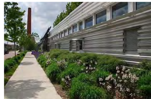
Example of separated, accessible walkway.
