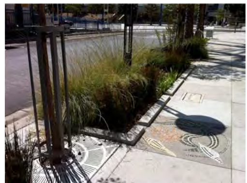
Example of a bioswale.
