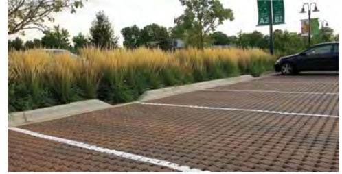
Example of permeable pavers.
