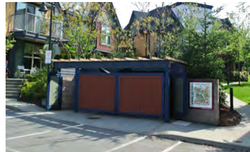
Example of screened waste enclosure.
