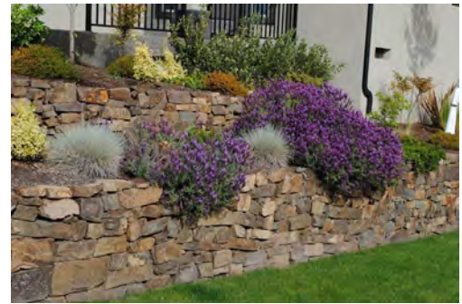
Example of stepped retaining wall.
