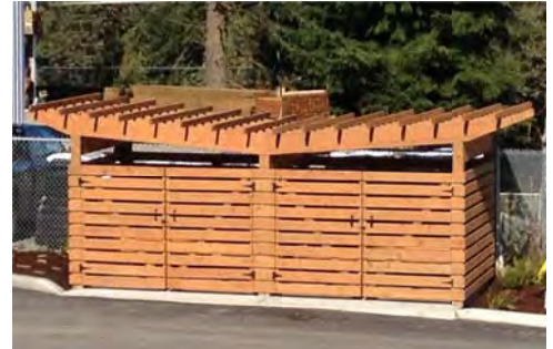
Example of screened waste enclosure.
