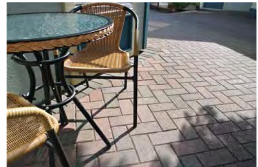
Example of permeable pavers.
