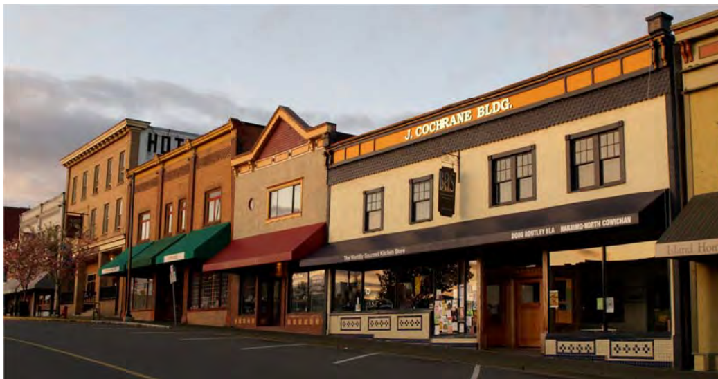
Iconic west side of First Avenue.
