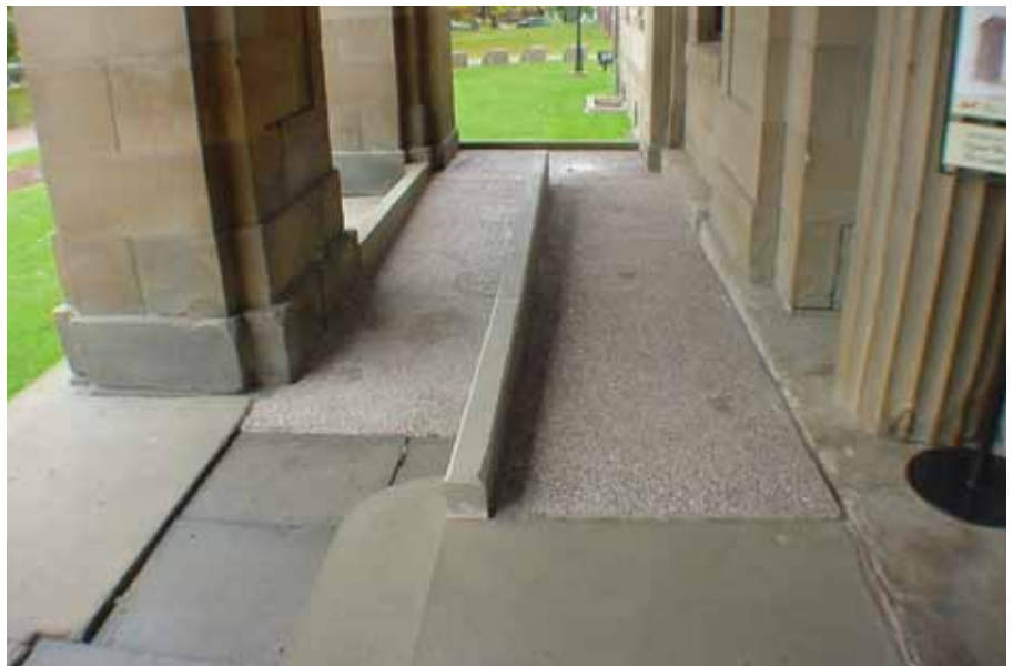
Adding a ramp to meet accessibility requirements should be designed to be compatible with a building's character. This new ramp at Province House in Charlottetown was discretely integrated into one side of an existing entrance porch.
