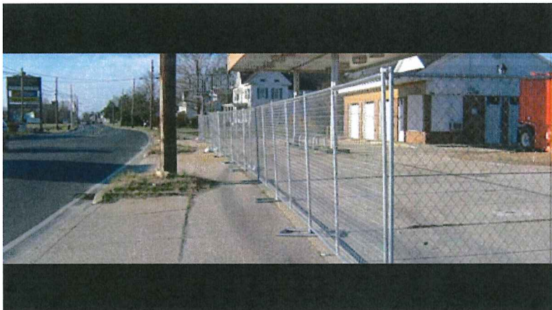
Figure 2: Temporary Fencing to be installed at 1030 Oyster Bay Drive
