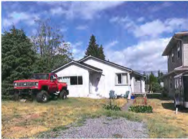
Figure 1: Existing frontage of 332 Warren St
