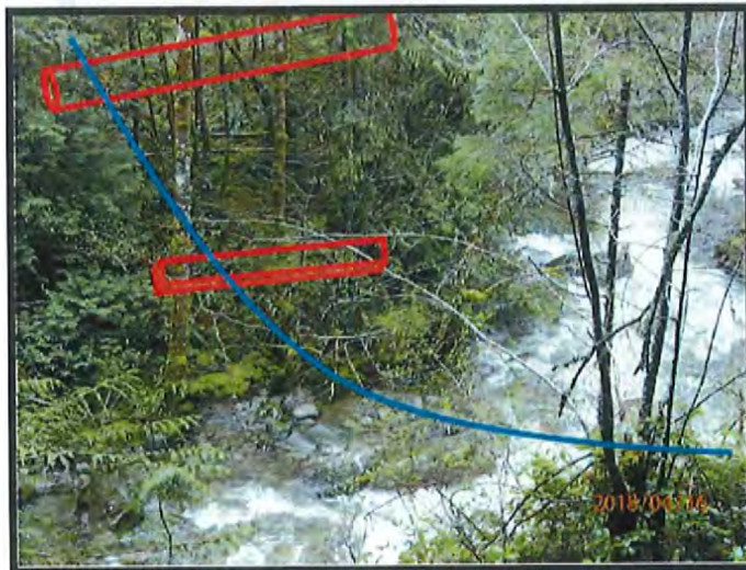
Photo 5. West ped pipe, footing and roadway. View is from east side of creek south (upstream) of structure.
