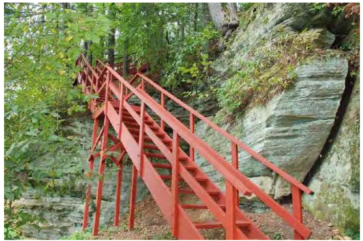
Connections such as staircases should be memorable and contribute to unique sense of place.
