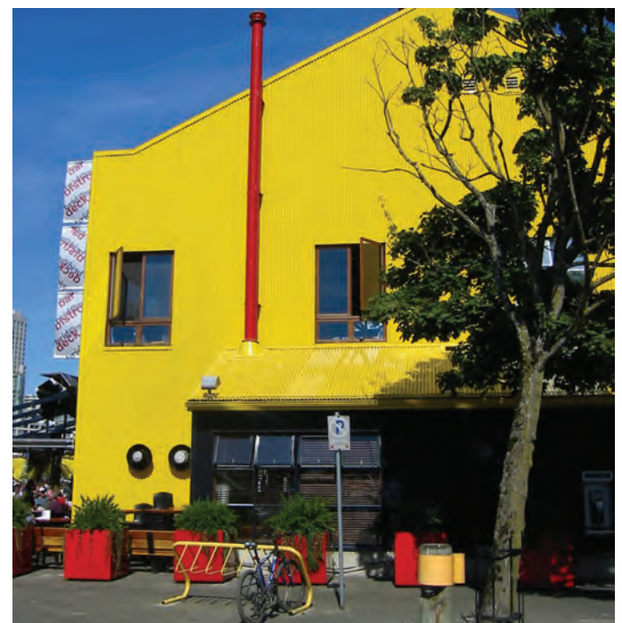
Example of a new building that uses corrugated tin cladding to complement historic industrial uses.
