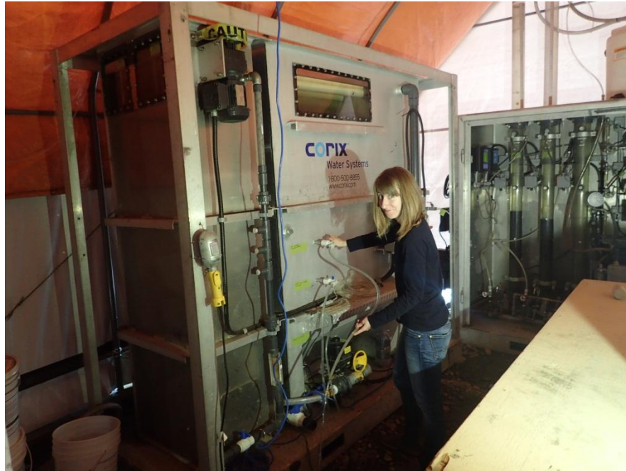
Settling Tank Skid
