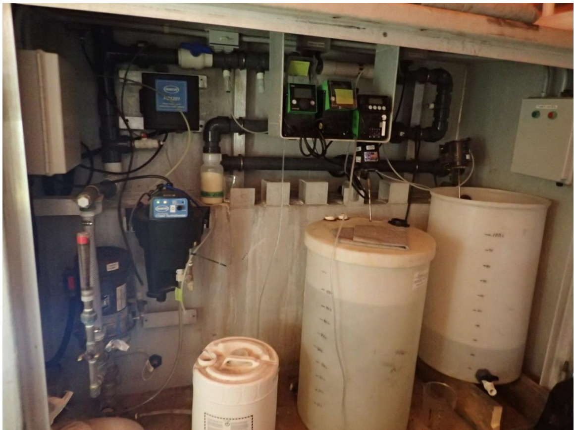
Chemical Dosing Skid
