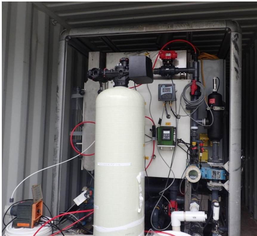
Membrane Skid in Trailer
