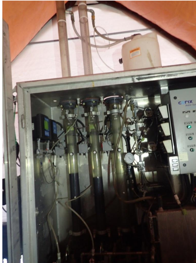
Media Filter Column
