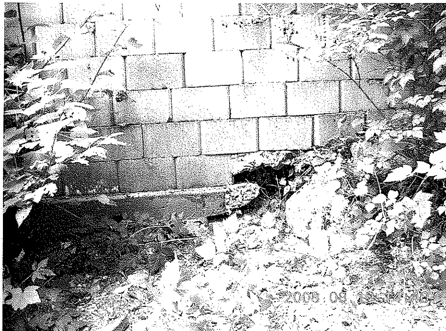
Photo 6: Void at toe of western approach retaining wall.
