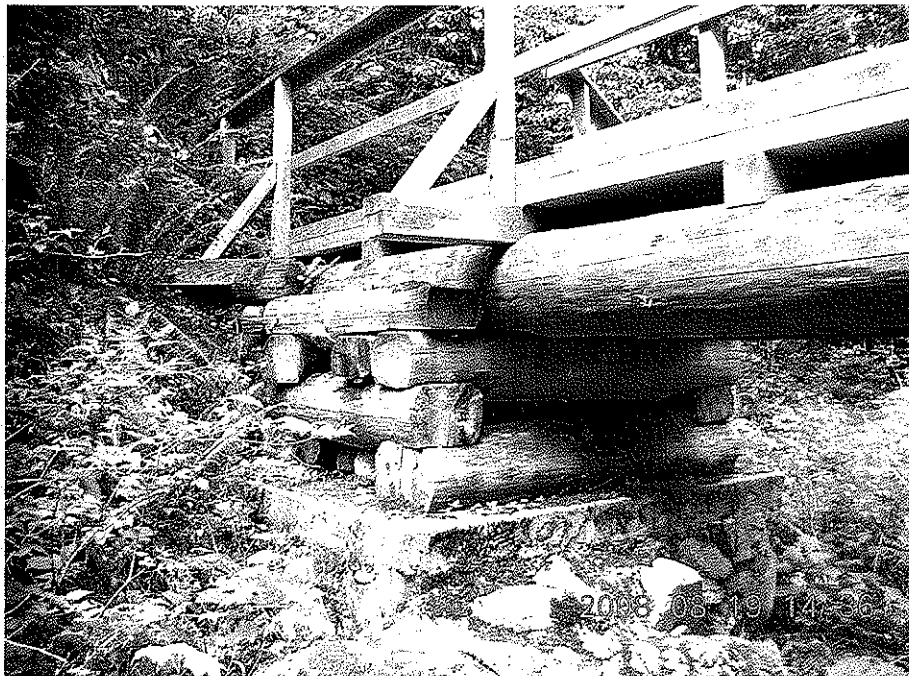
Photo 8: Rock filled log crib at the west end of the main span.
