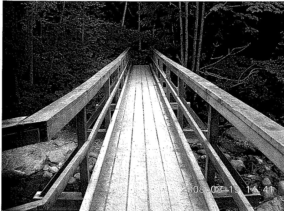
Photo 2: Main span looking East
