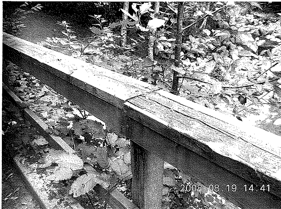
Photo 4: Cracked and splintered handrail.
