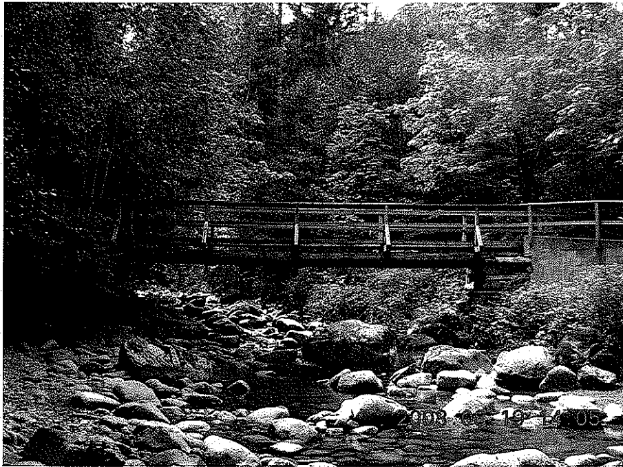
Photo 15: Main span looking upstream.
