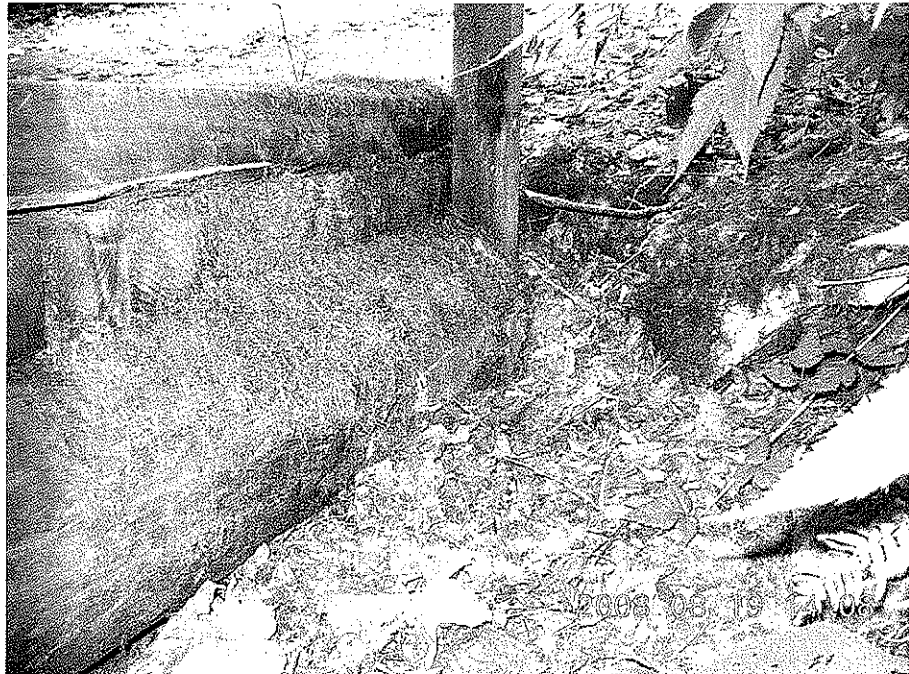
Photo 13: Eastern approach stringer in contact with ground.
