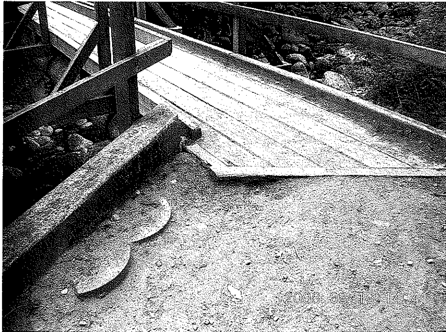
Photo 3: Top of western approach ramp showing tripping hazard
