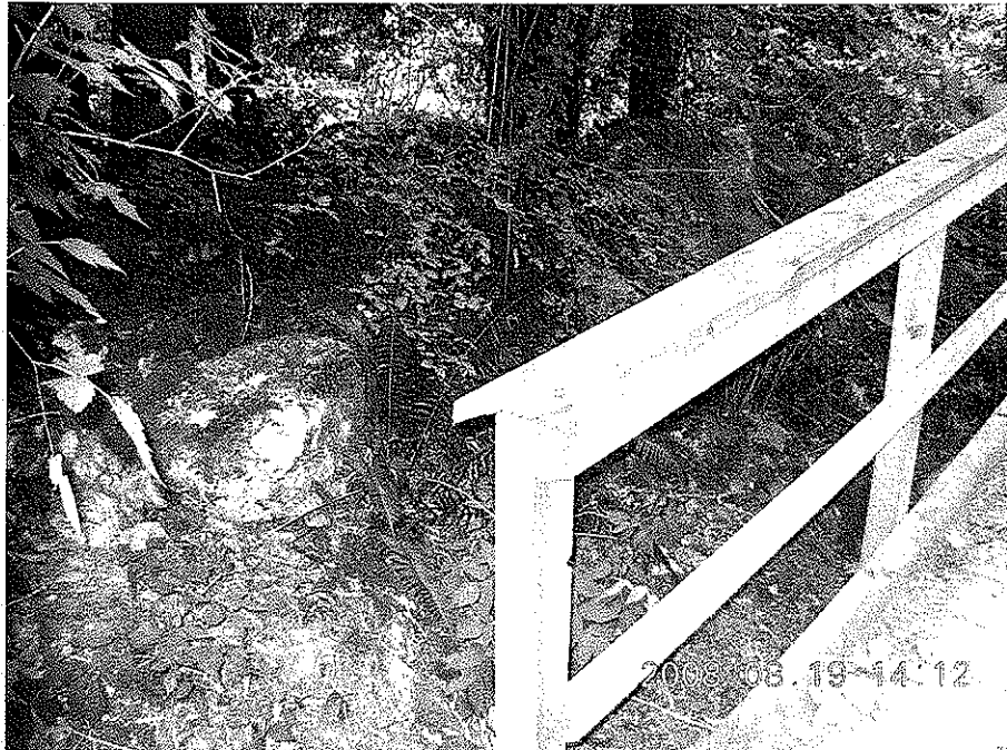
Photo 11: Handrail at east end of eastern approach broken off at end.
