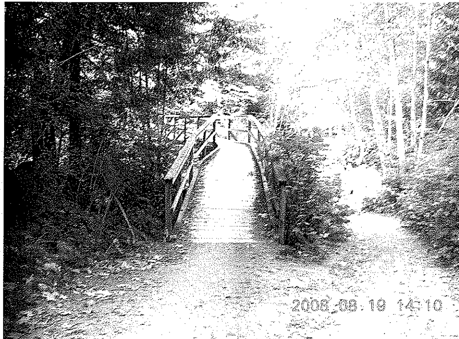
Photo 12: Eastern approach looking West.
