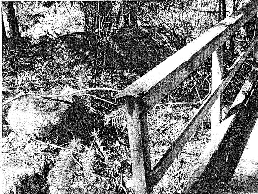
Photo 3: Handrail at Eastern Approach (note splintered end).
