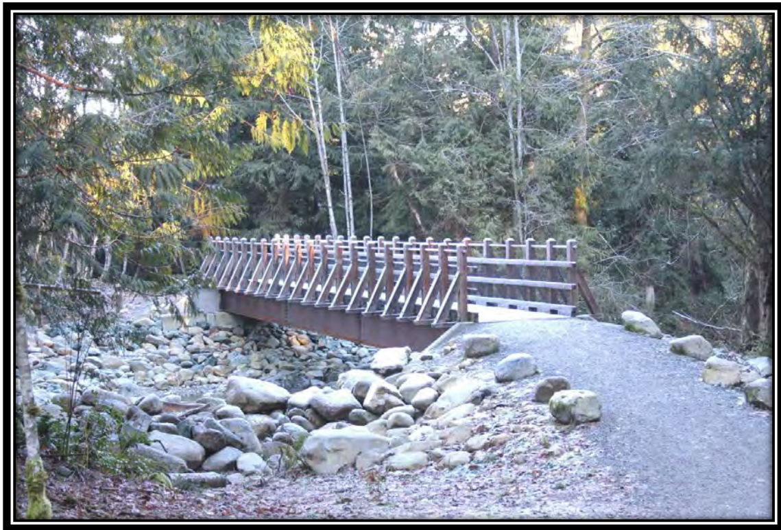
Holland Creek Pedestrian Bridge
