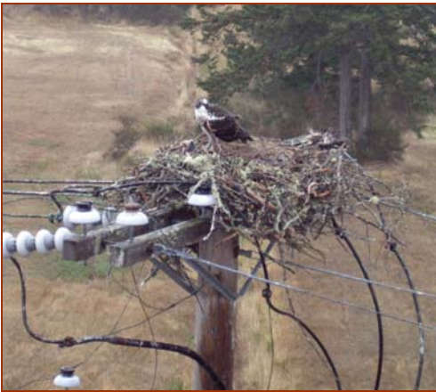
Figure 19. Ospreys commonly nest atop electrical poles and towers. Nests in such locations pose hazards to the birds and often result in costly power outages. LGL Limited photo.
