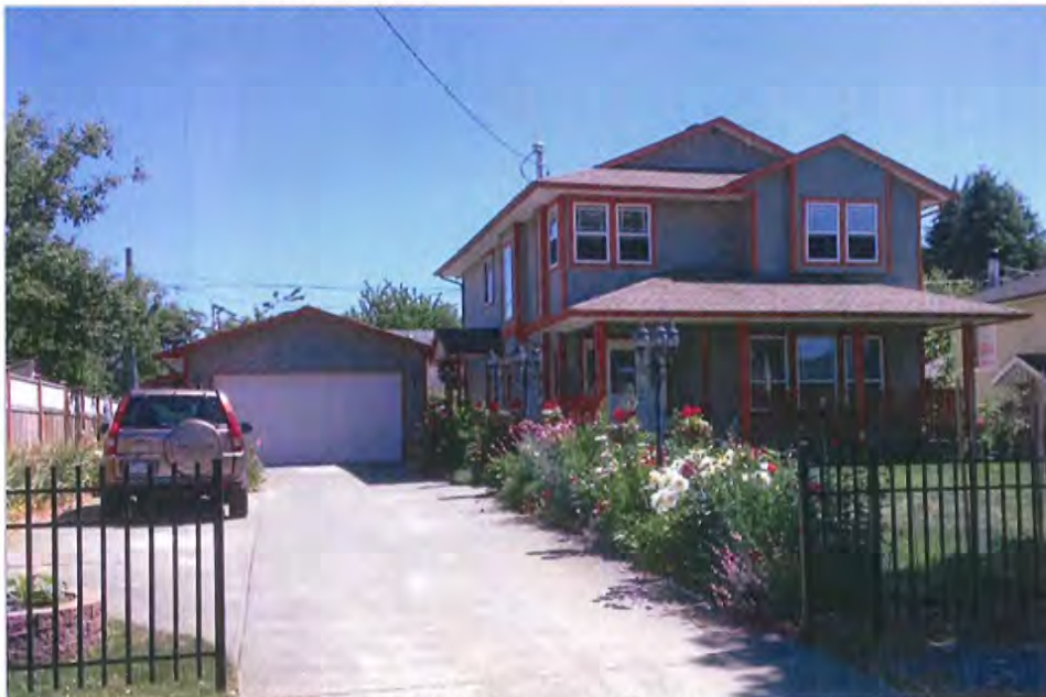
Photo 1: Accessory building at 509 French St. (view from French St.)
