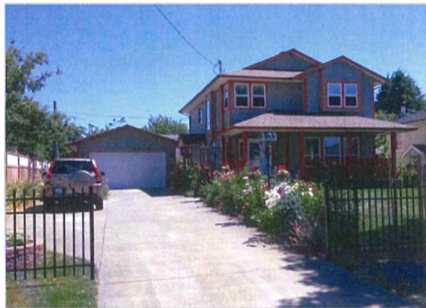
Photo 1: Accessory building at 509 French St. (view from French St.)
