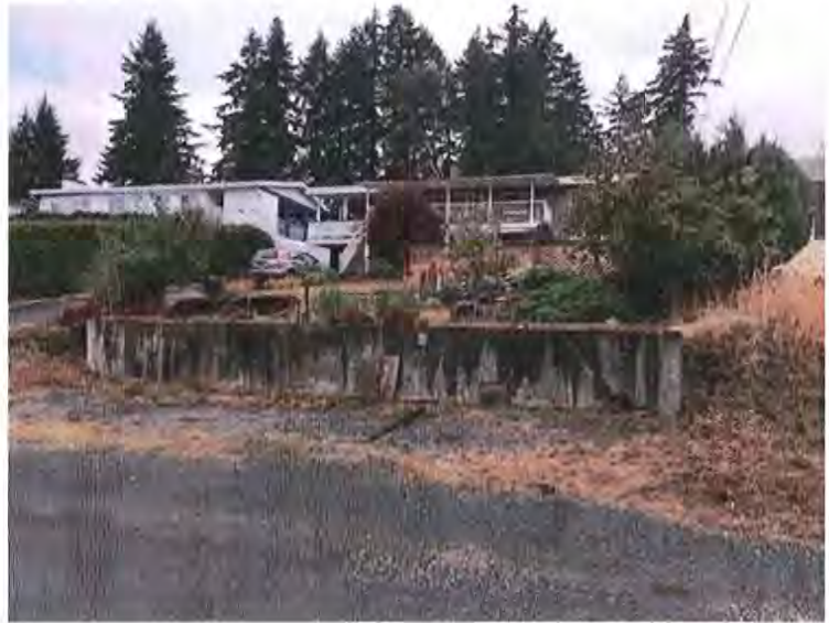
Figure 1: 1125 Third Avenue - View from the lane showing the proposed location for the coach house. The retaining wall shown in the photo would be removed.
