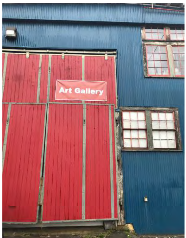
Existing entry door on South-East Facade
