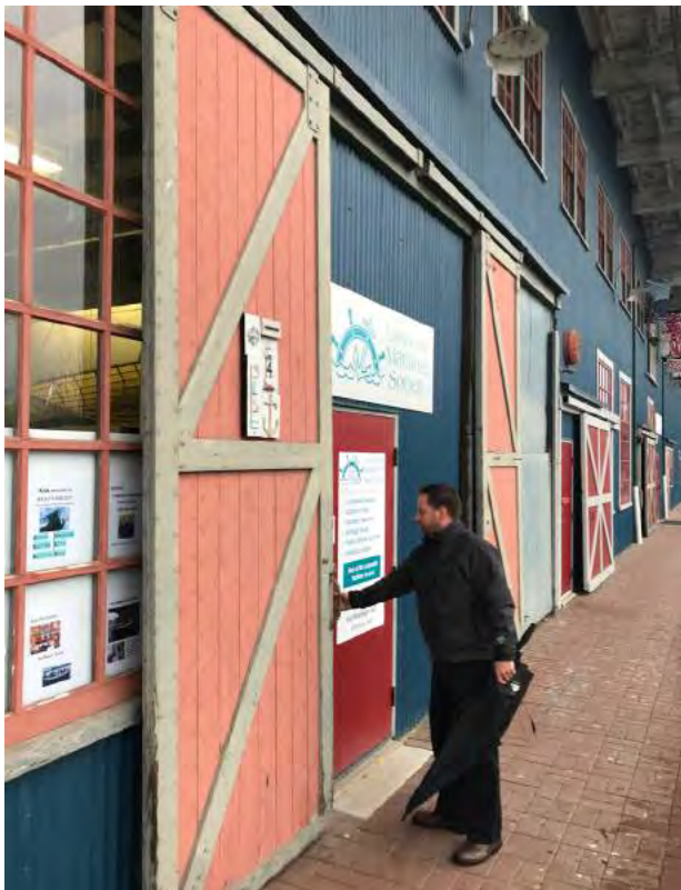
Existing entry door on North-East Facade
