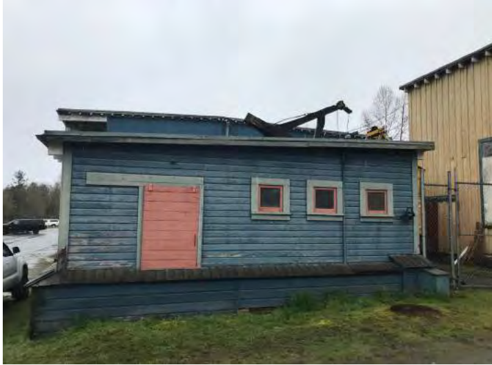
Existing adjacent building
