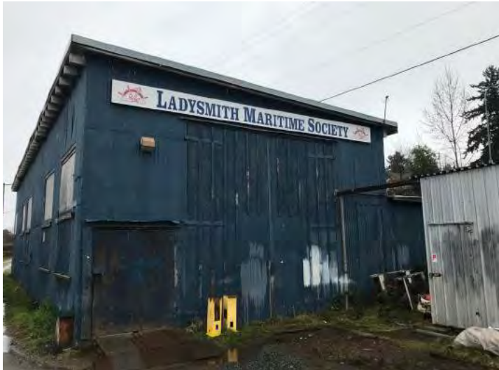
Existing adjacent building
