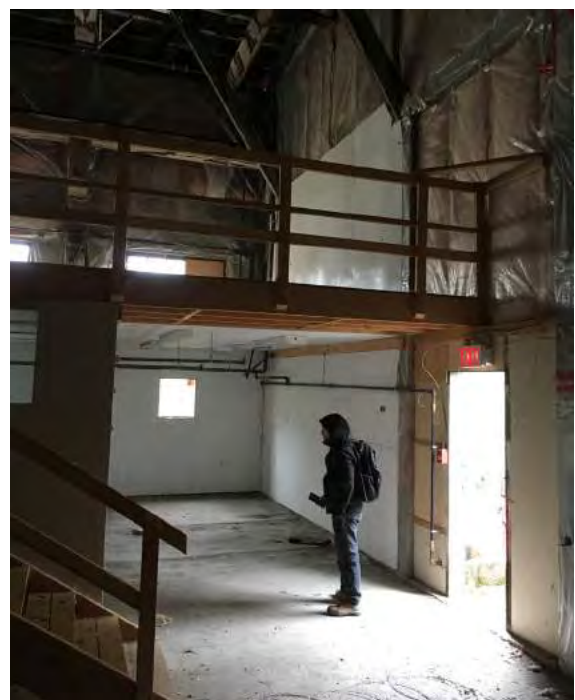
Existing Condition of Double Height Space
