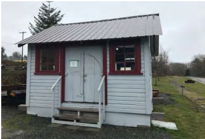
Existing adjacent building
