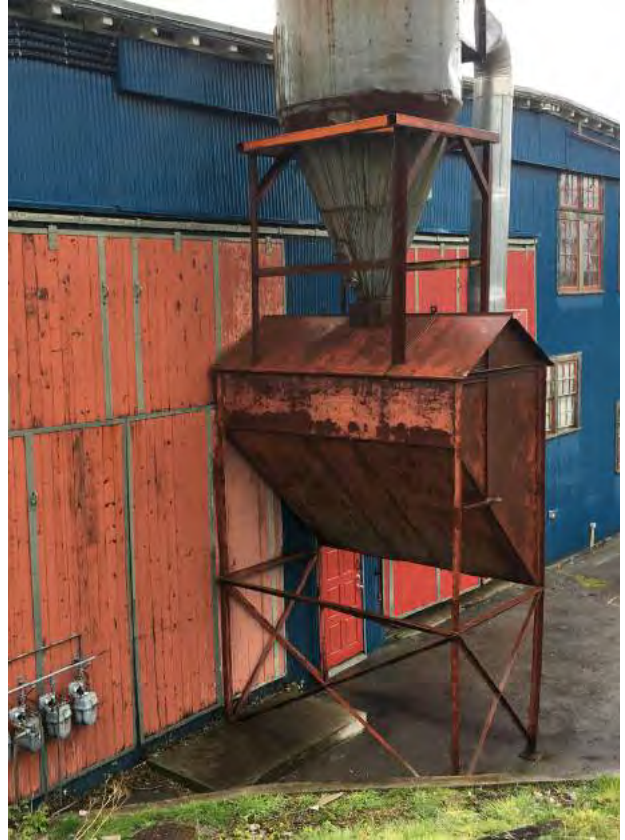
Existing South-East Facade
