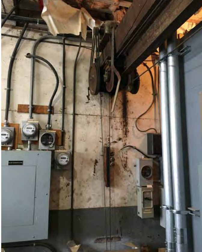
Existing Electrical Room
