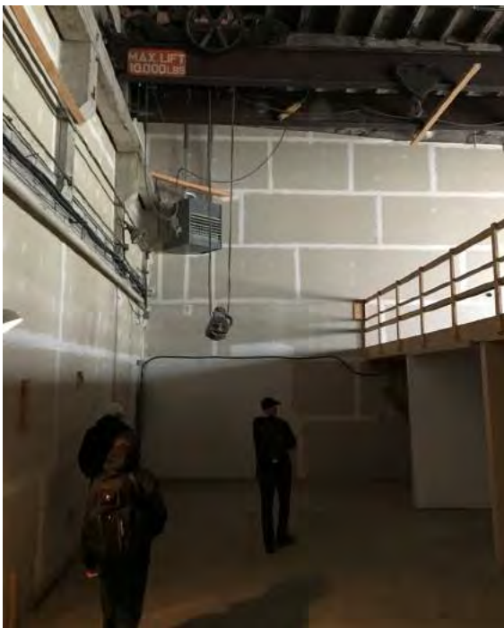
Existing Condition of Double Height Space
