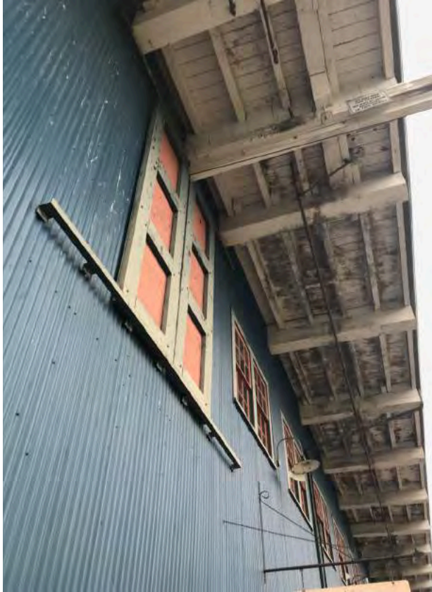
Existing soffit on North-East facade
