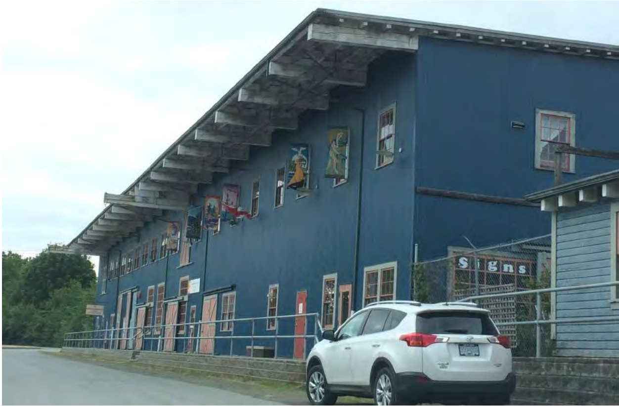
View of the front ("North" elevation) of the Machine Shop
