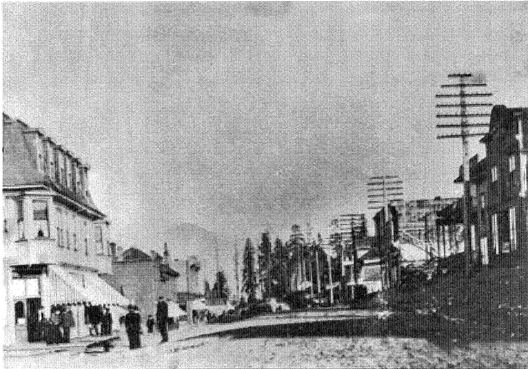
Construction of The Travellers Hotel – bottom right
