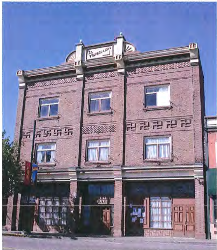
Photo 1: Front façade of vacant Traveller's hotel showing character defining elements.
