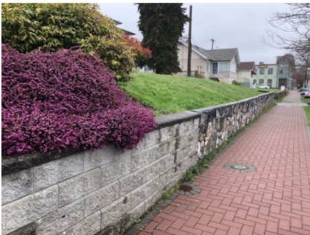
920 First Ave. retaining wall to be replaced to match 910 First Ave. wall as shown in photo above.
