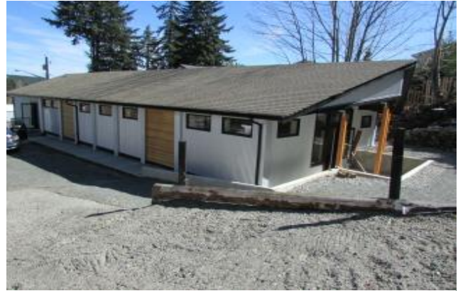
Photo 1: Existing building on the subject property at 1134 Trans Canada Highway.
