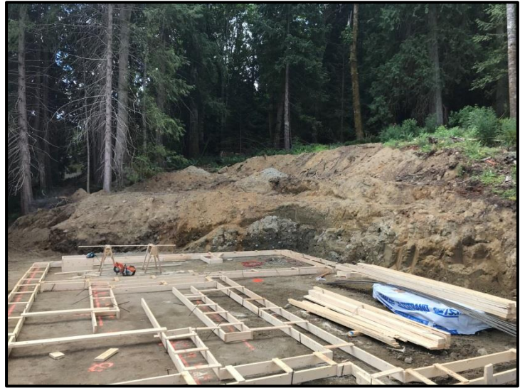
Dwelling under construction at 120 Kinsmen Place
