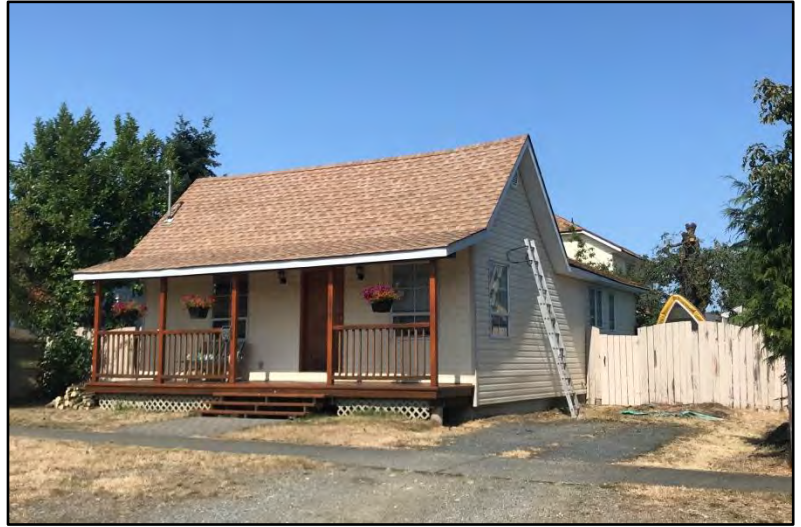
Street view of 420 Gatacre Street
