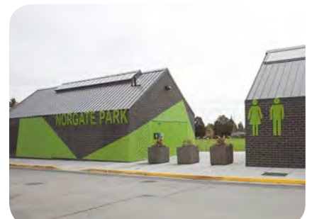
Park Service Building (carscdden.ca)
