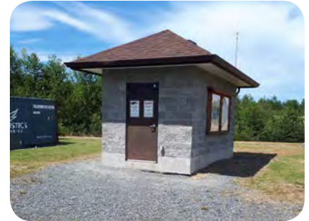
Electrical Building (LEES+Associates)
