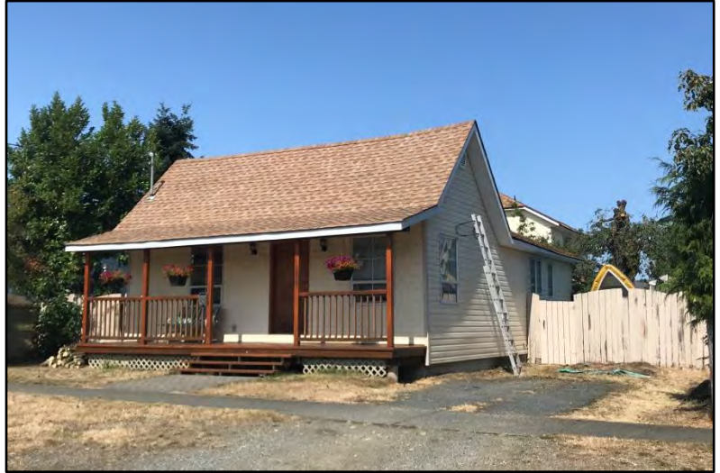
Street view of 420 Gatacre Street.
