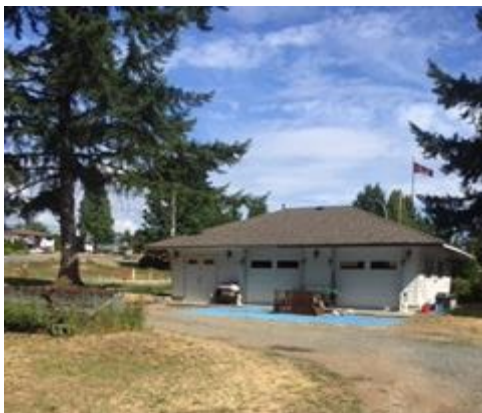
Figure 1: Existing garage - 341 Dogwood Dr.
