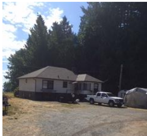
Figure 2: Existing house - 341 Dogwood Dr.
