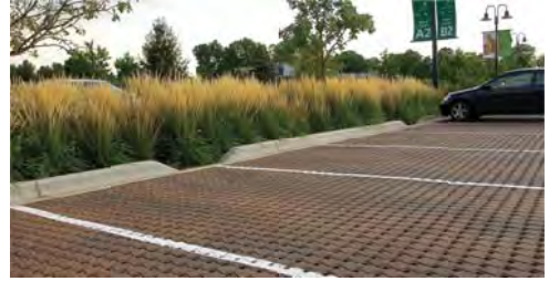
Example of permeable pavers.
