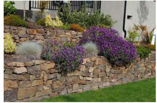
Example of stepped retaining wall.
