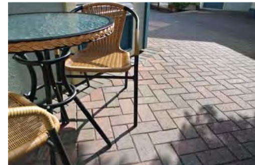
Example of permeable pavers.
