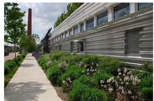
Example of separated, accessible walkway.
