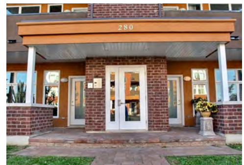
Example of weather-protected entrance.
