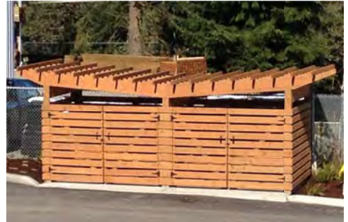
Example of screened waste enclosure.
