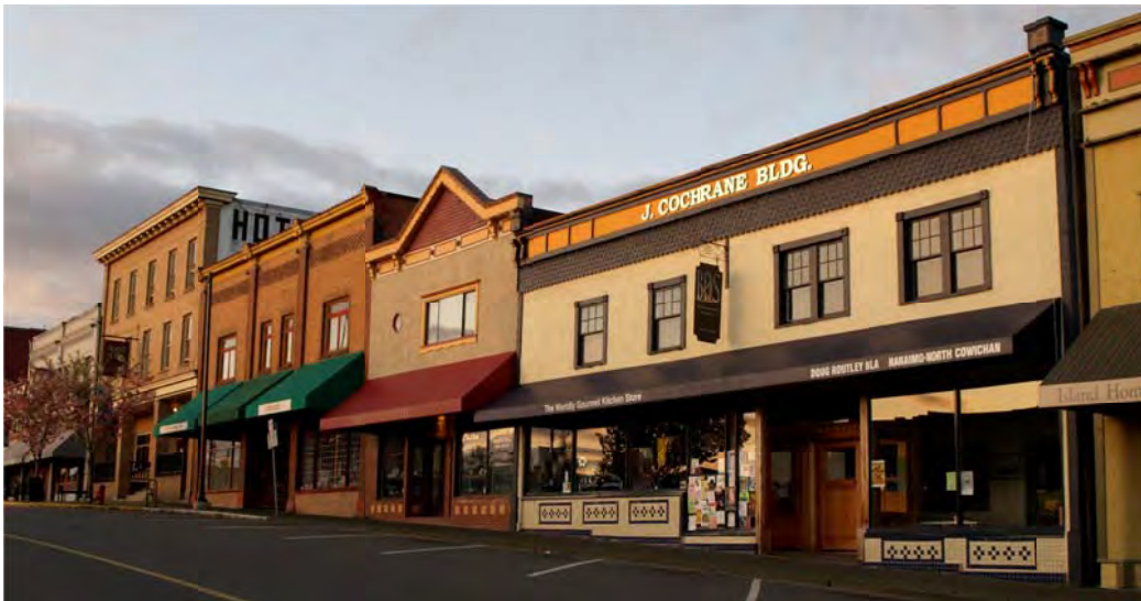
Iconic west side of First Avenue.
