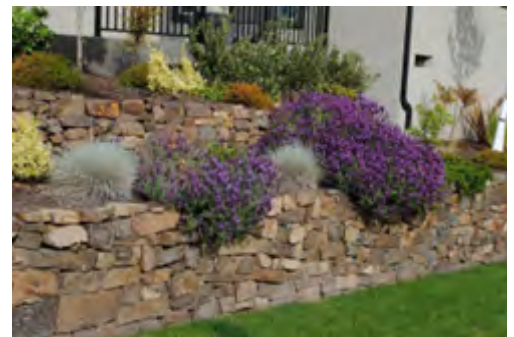
Example of stepped retaining wall.
