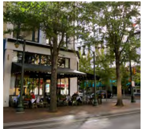
Example of high first floor ceiling height.
