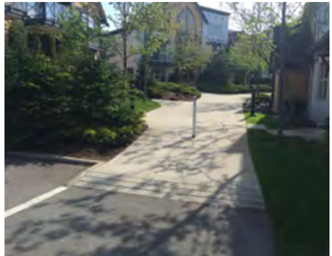
Example of an accessible curb.
