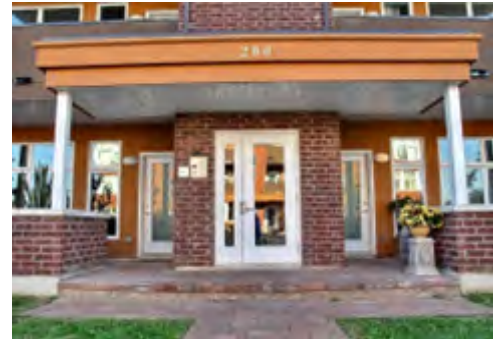
Example of weather-protected entrance.
