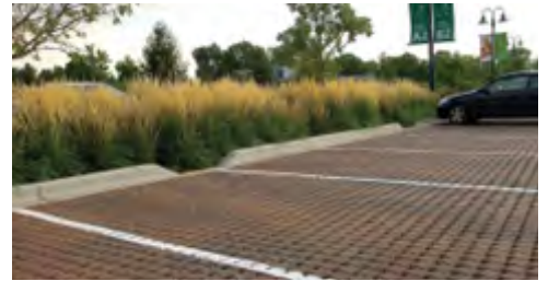
Example of permeable pavers.
