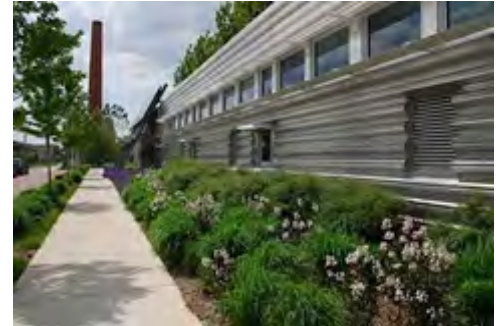
Example of separated, accessible walkway.
