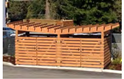
Example of screened waste enclosure.
