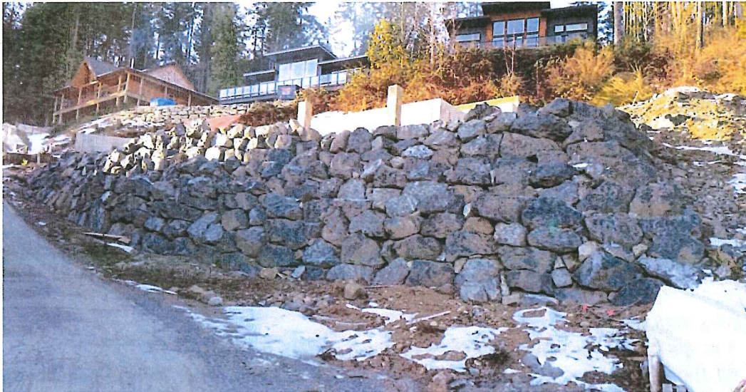
Photo 1: Rock retaining wall on east side of proposed house at 826 Craig Road
