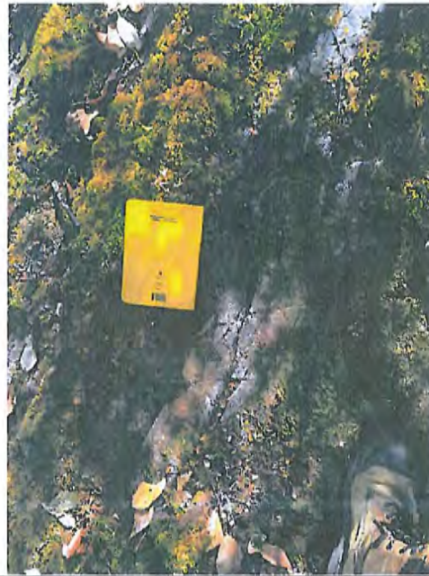
Photo 3: An example of the exposed bedrock, note fractures in the rock.
