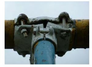
The swings are nearing the end of their service life. Although flaking paint is merely cosmetic, the dented support pole at the north end, and the bent bolts and possible shifting at the top caps/clamps of the south swings are of immediate concern. The safety zone for the swings meets current CSA Playground Safety Standards.
