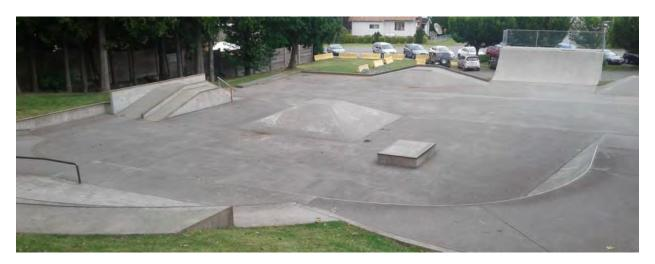
The skate park at Frank Jameson Community Centre is made up of a series of concrete ramps, steps and metal rails. Most of the concrete is in good condition, but there are some sections with hairline cracking to monitor, and some minor patching of chips and cracks needed. The fence at the top of the east ramp is curling up, and would benefit from additional ties and tension wires. Also concrete around metal coping needs patching in a few spots.
