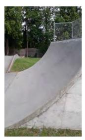
There appear to be a few design and flow issues with the structures as they are. The south side ramp is not well-used, as evidenced by the good condition of the fencing. The transition from pyramid at the base is a sharp 120 degree angle, which limits flow onto and off from the feature. Also, the drop in to the half pipe is steep and has a sharp curl at base that could be difficult to negotiate. Finally, the grinding rail at the east side appears to be a little high.
