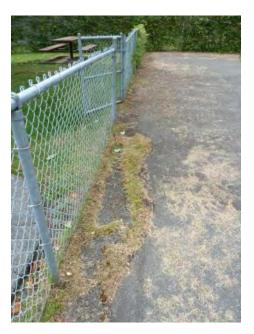
The chain link mesh at the north corner is bowing out due to the lack of a tension wire at 3' height. Mesh is also damaged along the top rail of the south section, but does not currently present a hazard. The neighbour is growing wisteria vines along the south fence, which provides some whimsy to the park, but may restrict future fence repairs or replacement.
