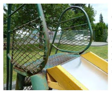
The slide is an older metal frame style made by Blue Imp. It faces southeast, which is not a preferred aspect due to heating from the sun. Although the welds on the slide are in good condition, there is an area at the top corner of each side that may present an entanglement hazard. This style of slide no longer conforms to current standards.
