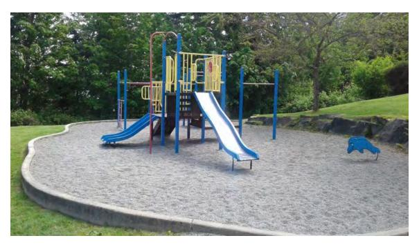
This playground consists of a Blue Imp platform structure connected with monkey bars, rings, and chinup bars, plus a small dolphin bouncy rider. The concrete border is in good condition, with only a few small chips in the cap. The pea gravel is a little finer texture than pea gravel at other playgrounds, but it appears adequate for the height of these structures.
