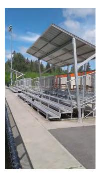
Chain link fencing is good quality, with 9 gauge black vinyl coated fabric, a tighter weave and more frequent ties. Top rails have areas where paint has flecked off the galvanized surface underneath. The aluminum bleachers are of good quality, with only occasional maintenance required to inspect and repair the chain link backing, particularly where the bottom edge may start to curl in.
