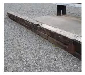
The creosote wood stringer retaining wall between the swings and other play structures is pushing outward, and top cap boards are uneven and breaking down at the end of their life. This wall could be replaced with a similar timber retaining wall. If the wall were to be removed, the two benches and pads along the top of the wall would also need to go. With no wall, additional pea gravel may be required to reduce the downhill migration from the swings to playground area.
