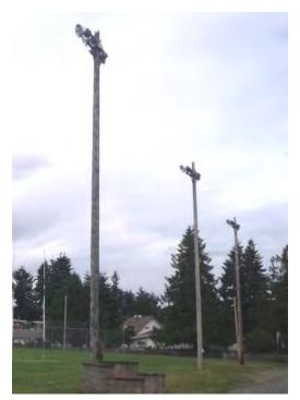
At the east end of the grass fields behind FJCC, there are three wooden poles with sports field lights. With 4 lamps per pole, and the low height, these lights would provide practice level field lighting to a portion of the field.
