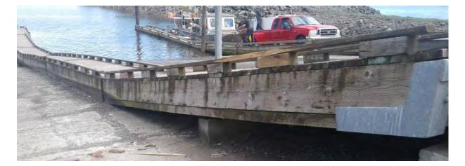
The decking and substructure on the floats is made from pressure-treated wood and is in fairly good condition. There are few slightly loose boards, but they are not a hazard, and the substructure is still holding the nails from the decking well. The floats are a good design and have a life expectancy of 15-20 year with proper maintenance. Three new metal pylons were installed in summer 2017.
