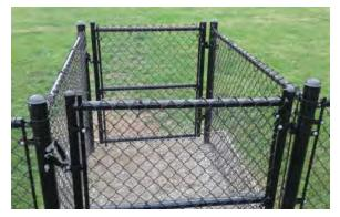
The chain link mesh is only 9 gauge vinyl, which means the wire inside is only 12 gauge. There is a top rail, but with ties roughly only every 10 knuckles, and a bottom tension wire instead of a rail, the fencing is prone to damage from contact with people or equipment.
