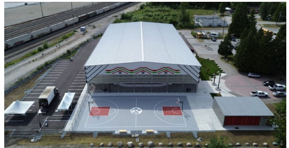
The Squamish Nation's Kw'eshkw'shétsuta'y
