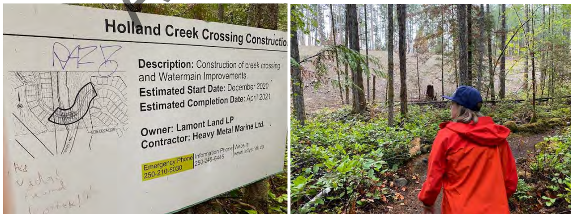
Left: Holland Creek Crossing Construction. Right: View from Holland Creek trail to construction area.
