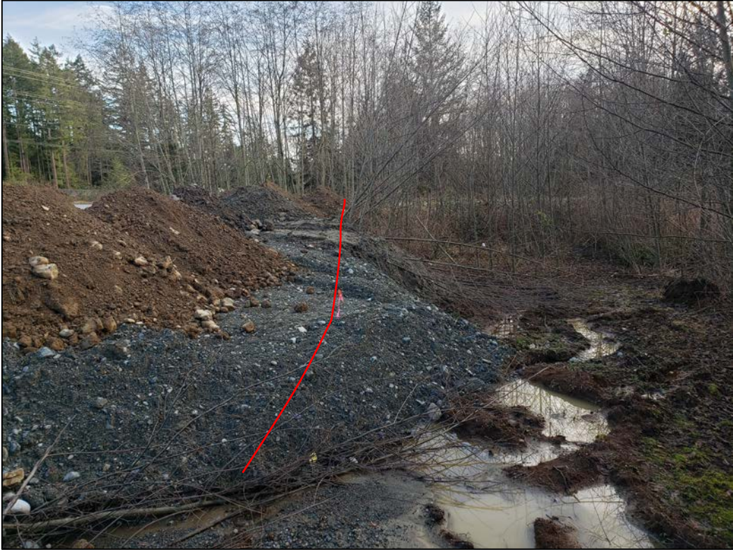
Photo 3. Showing a portion of the fill within the 15m SPEA looking toward Westdown Road.
