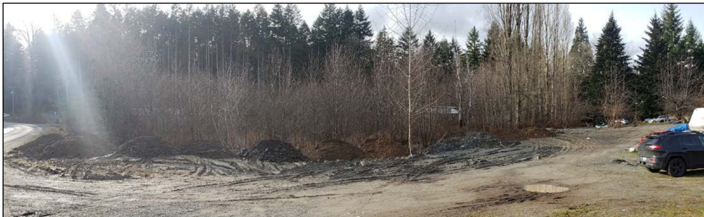
Photo 2. Showing the same view where the fill has been placed in the 30m DPA of Kerr Creek up to the row of red alder trees.
