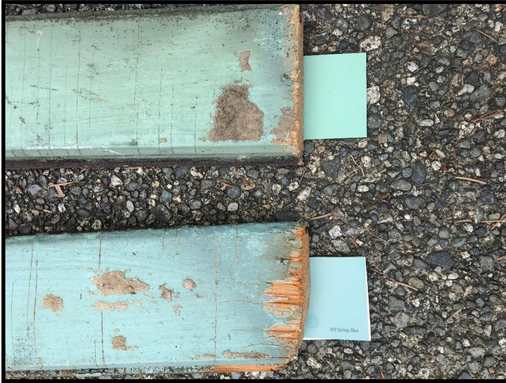
Figure 1: Options for paint colour for main siding. Boards were found on building and matched to available paint colours (top: Southfield Green, bottom: Mill Springs Blue, both Benjamin Moore).
