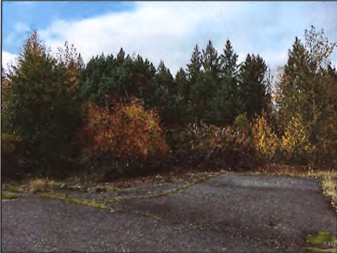
Photo 11. Showing one of many paved trailer pads that extend off the access roads.
