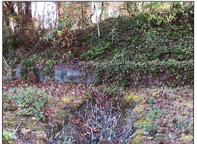
Photo 14. Showing an old cinder block retaining wall at the base of the slope leading up to Gladden Road.
