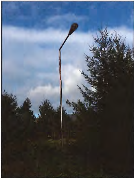
Photo 13. Old street light posts remain in the trailer park area.
