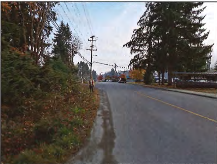
Photo 22. A roadside ditch is located along the east side of Rocky Creek Road that begins across from the Madill site and runs north.
