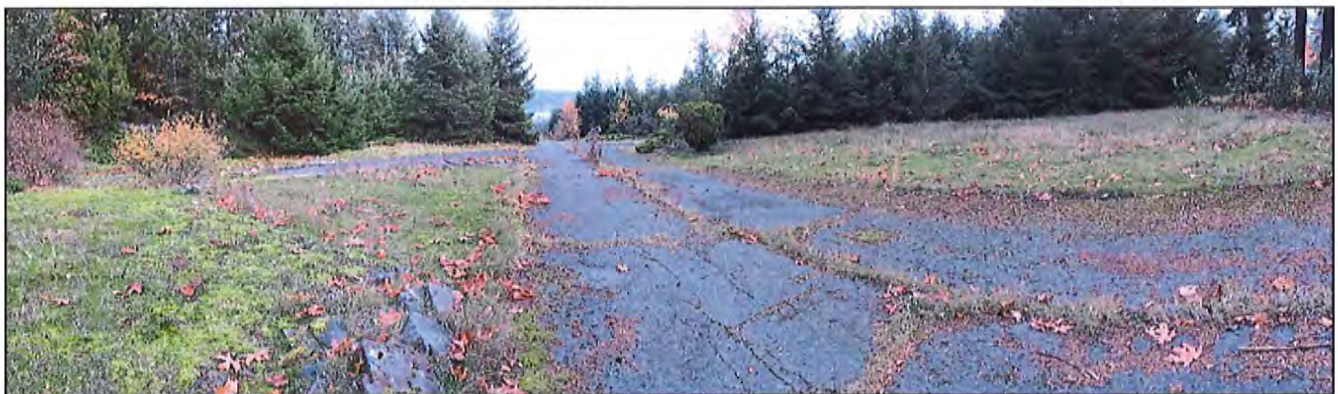
Photo 10. Showing the second of the two paved trailer park access roads.
