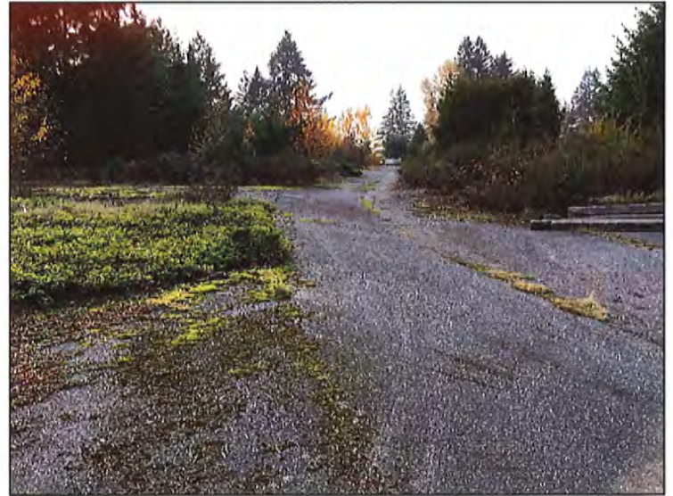
Photo 9. Two paved access roads with trailer pads bisect the centre of the 1301 Rocky Creek Road parcel.
