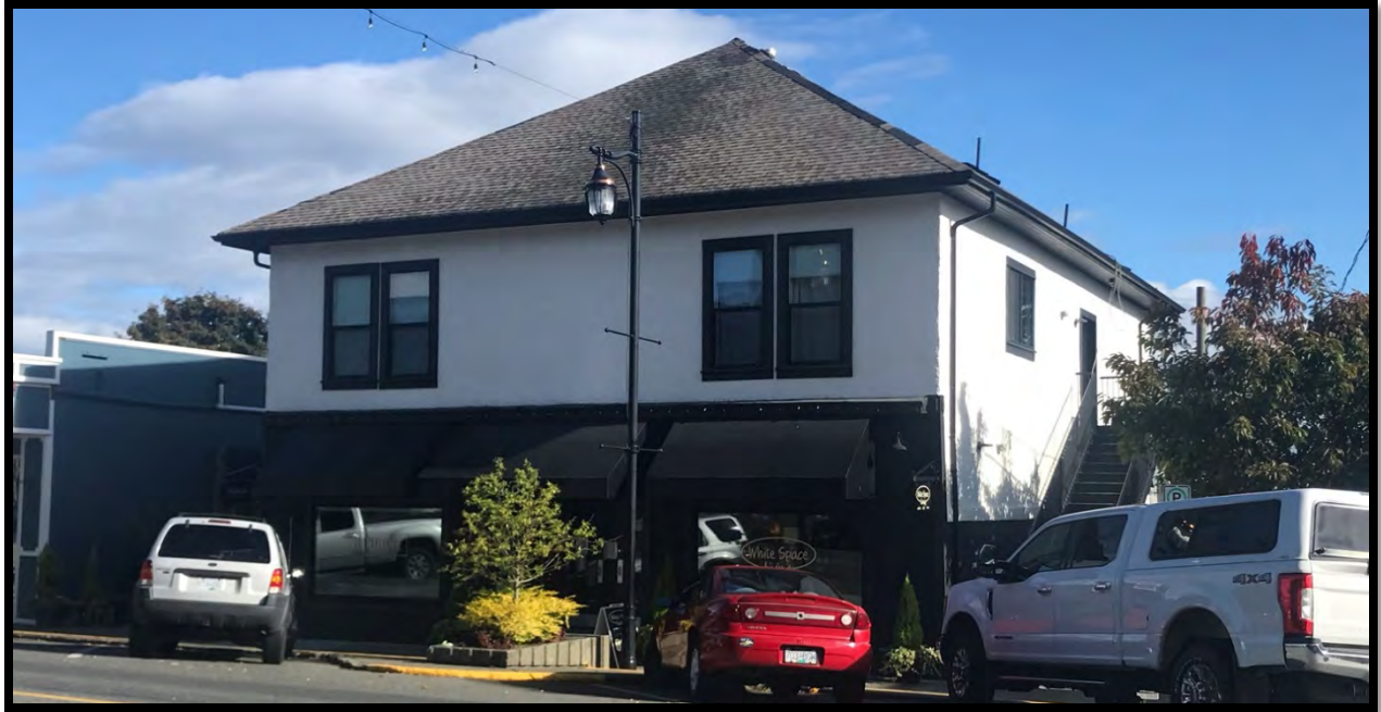
Figure 3 - Existing building at 431 1st Ave. Photo taken September 28, 2021.
