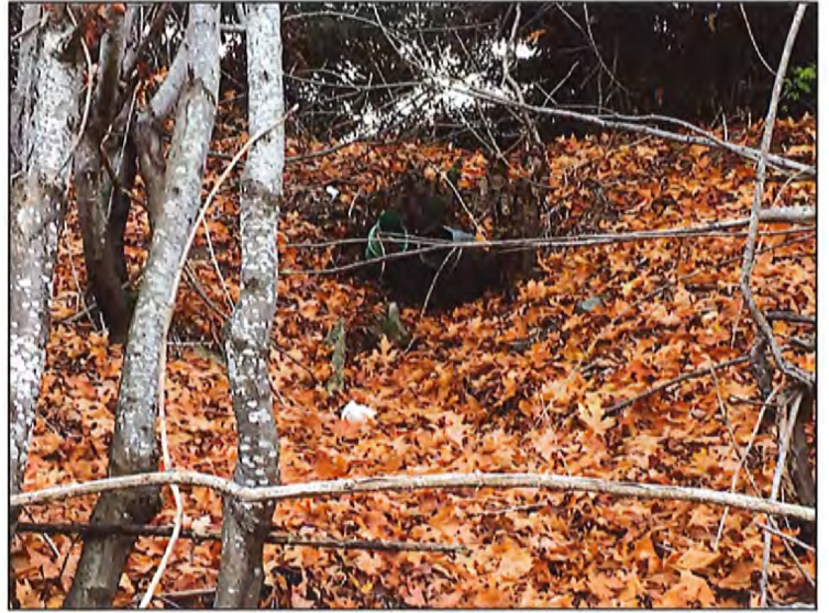
Photo 7. Two PVC drainage pipes near the top of the foreshore slope.
