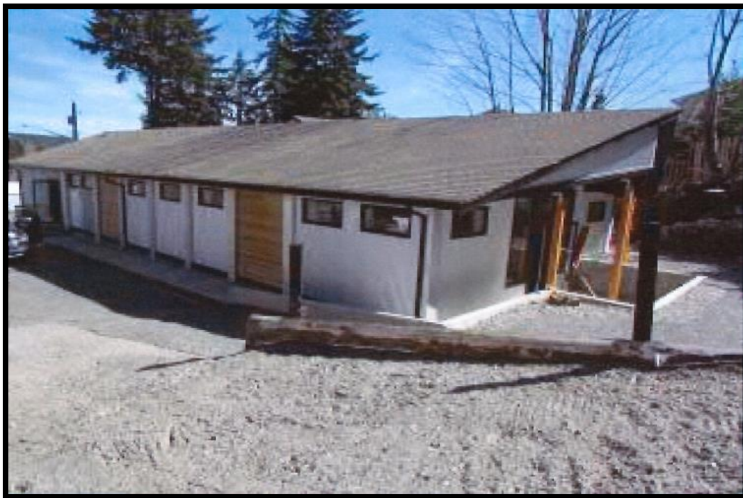
Figure 1: Existing Building 1134 Trans Canada Highway
