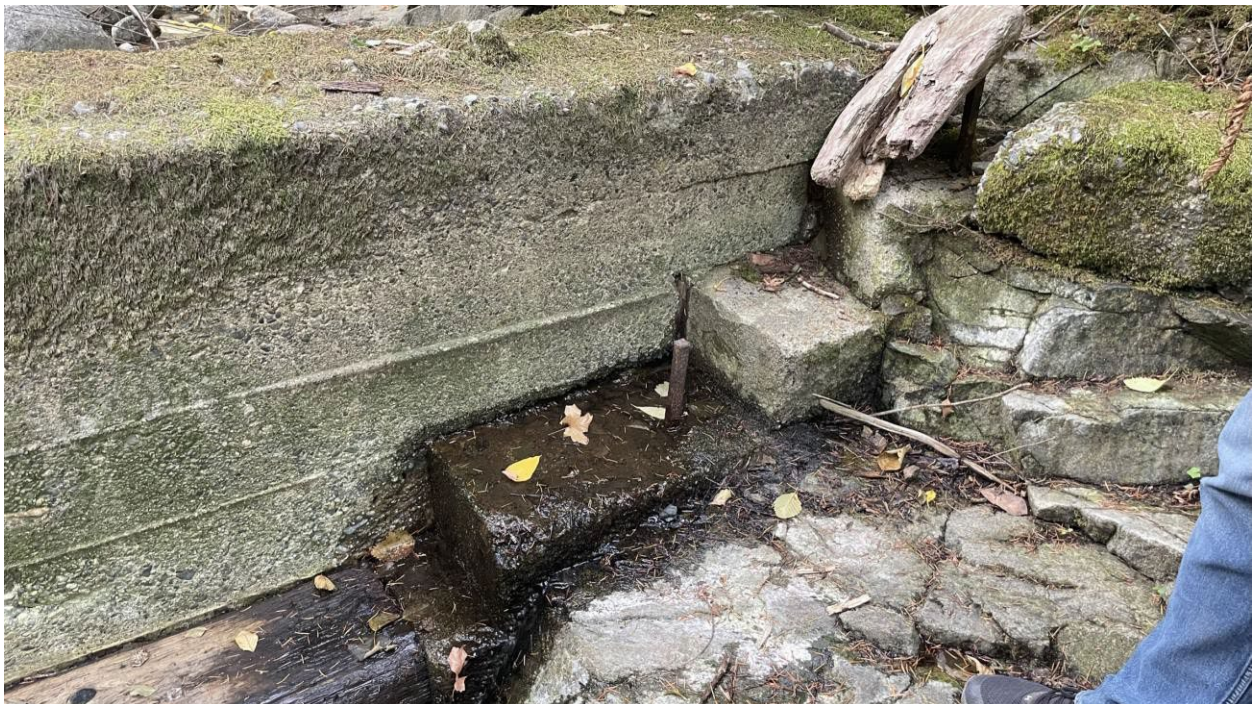
Photo 6 Seepage underneath left concrete abutment.
