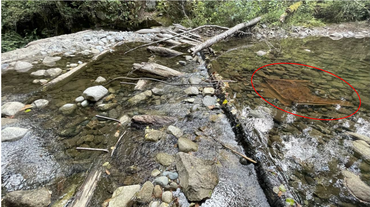
Photo 2 Low-Level metal intake grate and remnants of wooden flashboards, looking east (from left side of dam).
