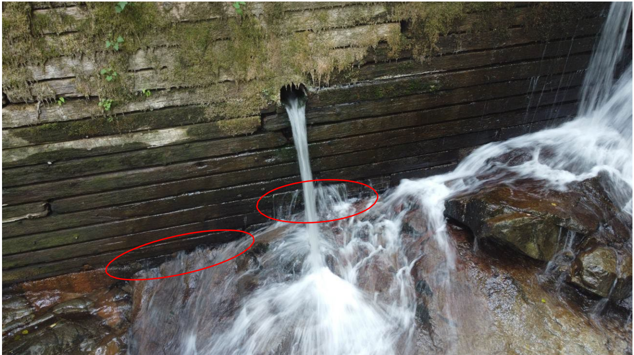
Photo 7 Major seepage at toe of downstream face.
