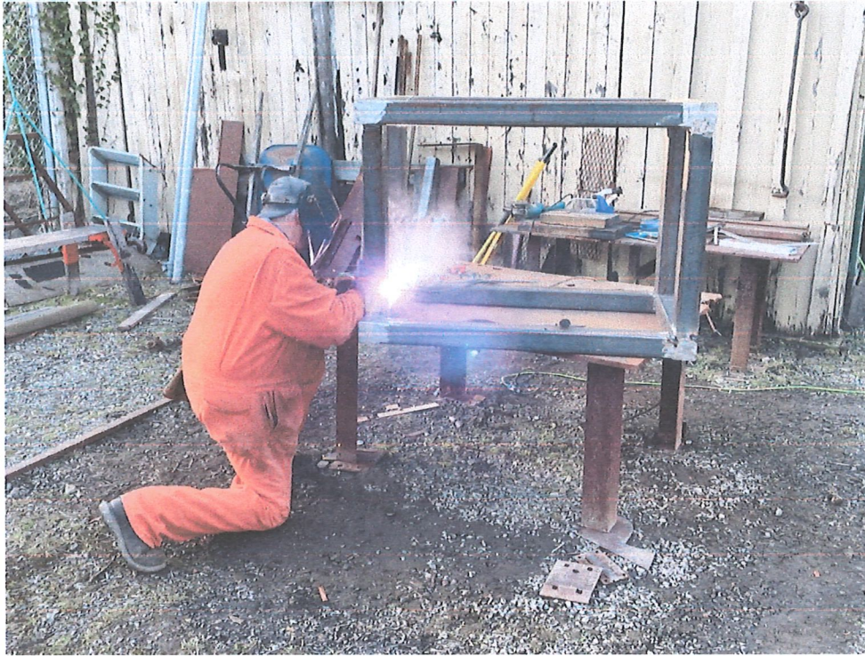
Fabricating the steel stand for the bell display
