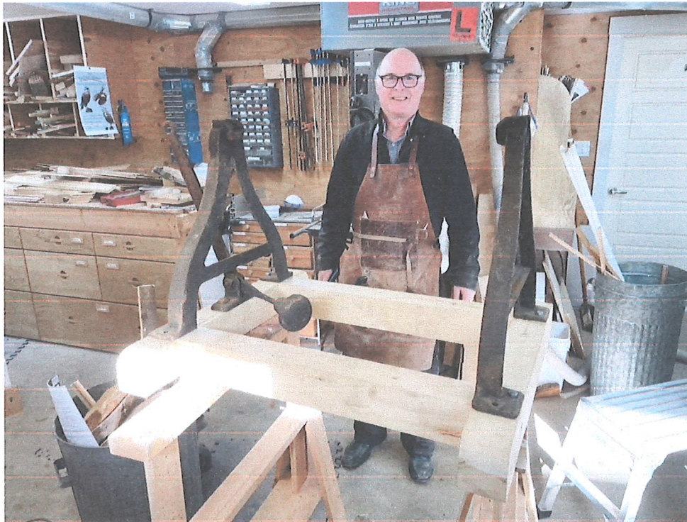
The rotten wooden bell crib was replicated in yellow cedar
