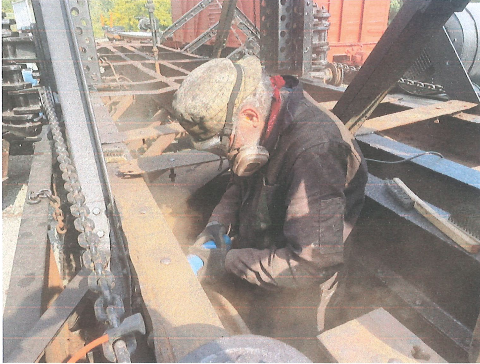
Descaling the rusted framework prior to rustproofing
