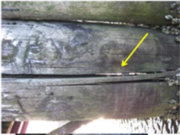
Severely split bearing pile
