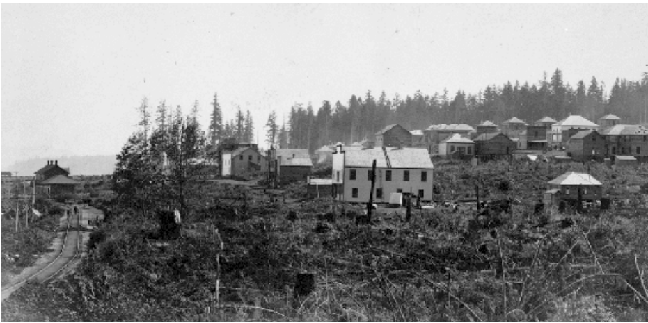
Ladysmith under construction (BCA c_03714)
